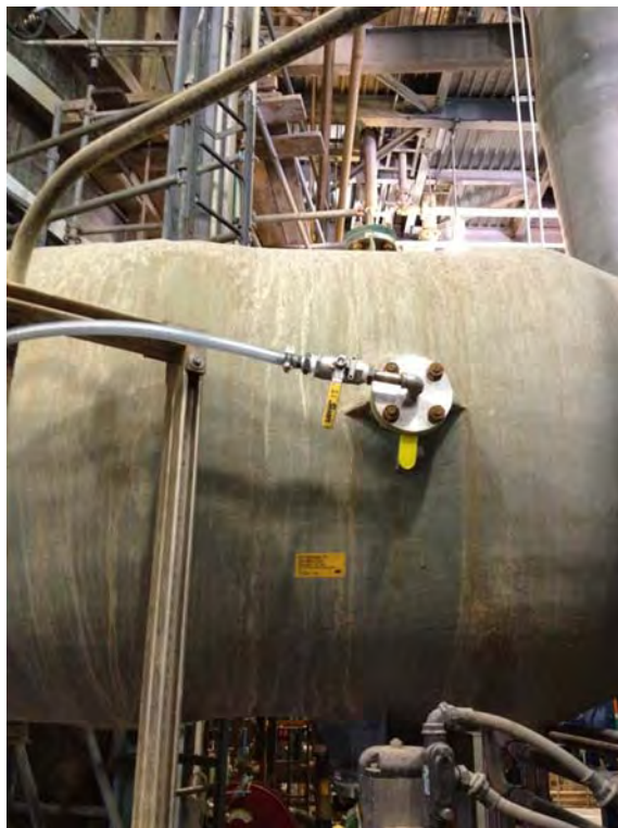
Recirculation Line Injection
